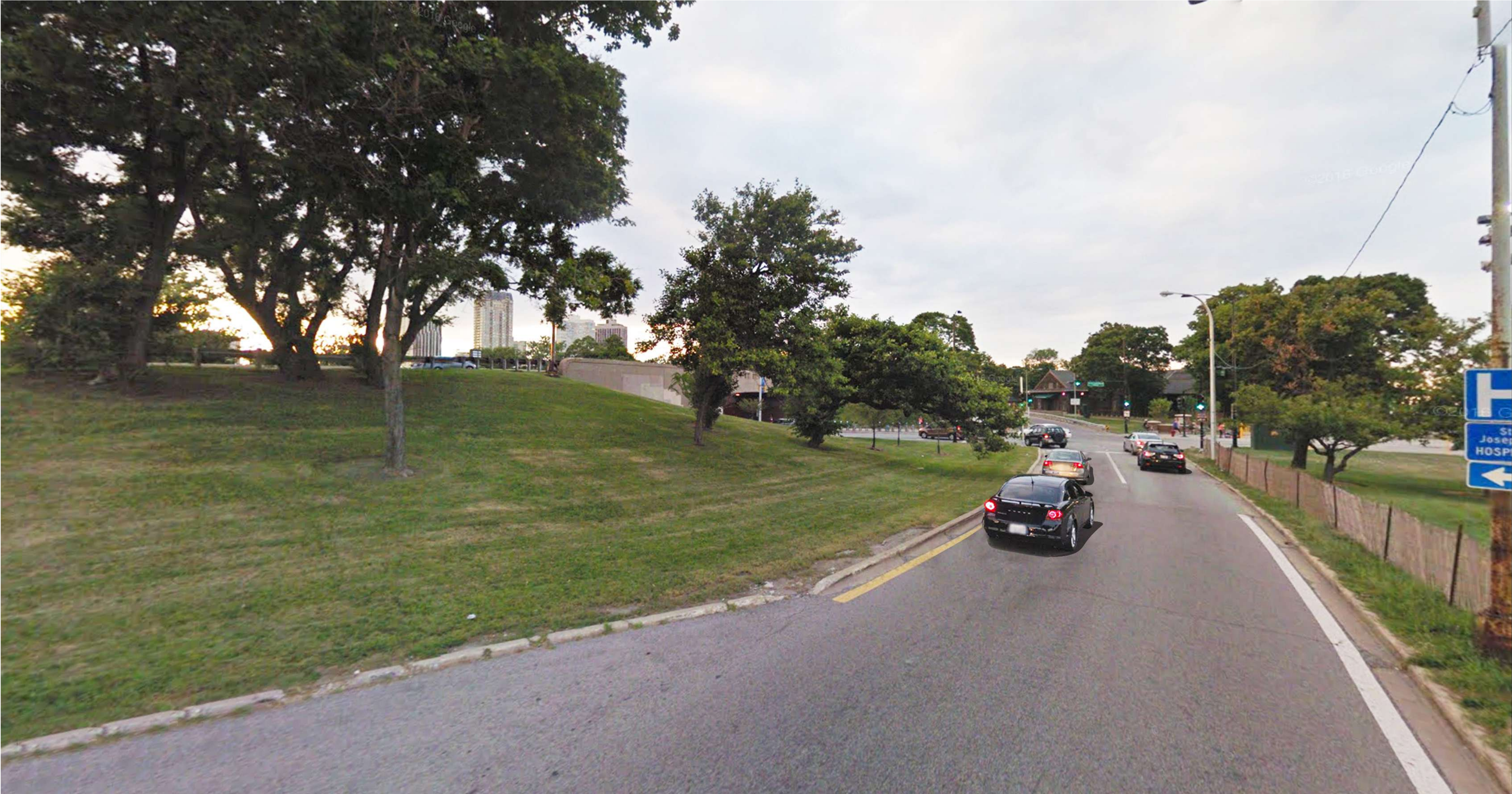
Typical Existing Junction with Grass Embankment - EXISTING VIEW
